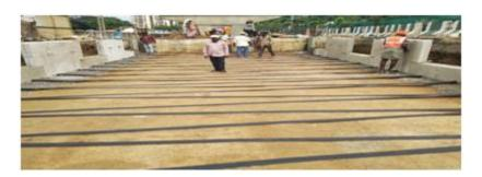
Fig.2: Shows Geo-textile Used in Road Work at Madhapur
